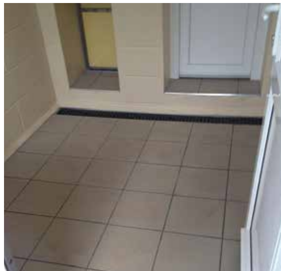
Internal cleanable flooring
